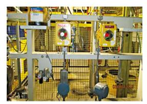
Fig. 4 Chemical flow meters
