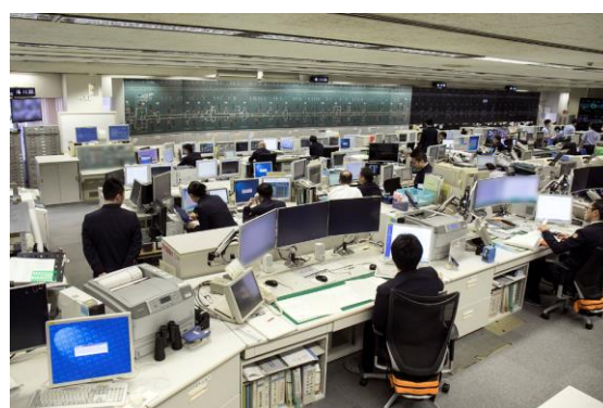
Shinkansen General Control Center
