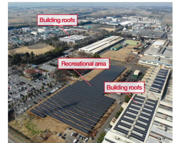
Panoramic view of the PV power generation system at the Moka site
