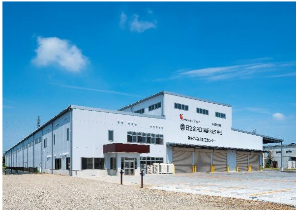
Hitachi Metals Tool Steel Eastern Japan Logistics Machining Center (Kazo City, Saitama Prefecture)
