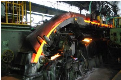
Continuous casting and rolling equipment
