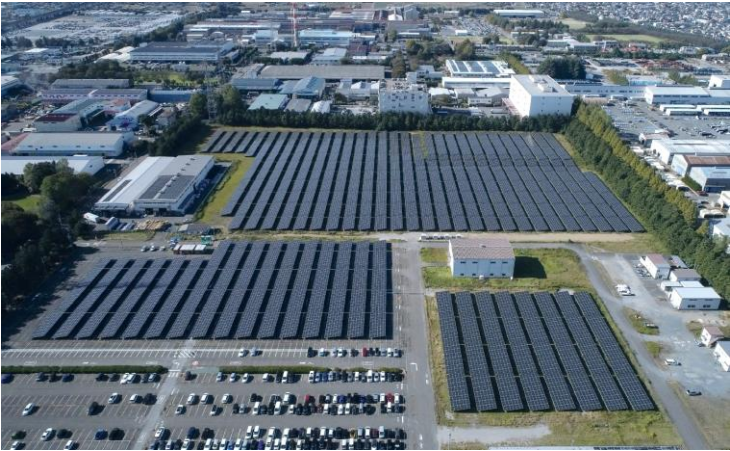
One of the largest off-grid photovoltaic power generation facilities in Japan (Kumagaya area)
