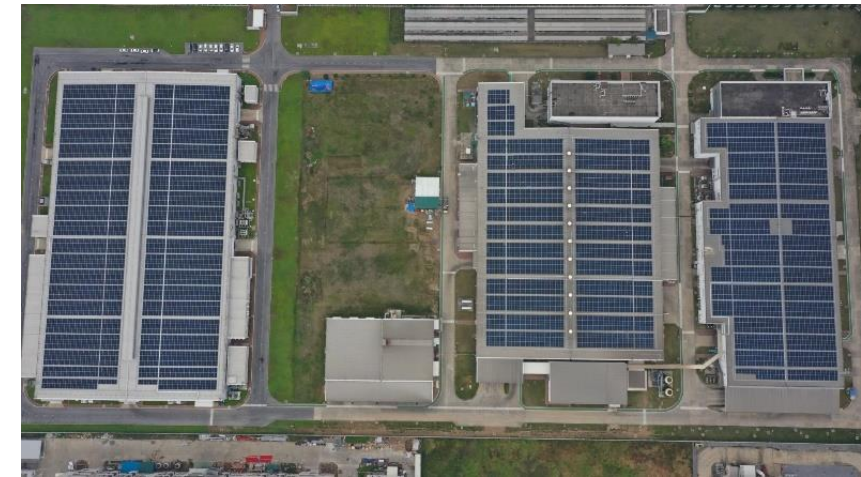
Bird's-eye view of the photovoltaic power generation facility (Proterial Vietnam)
