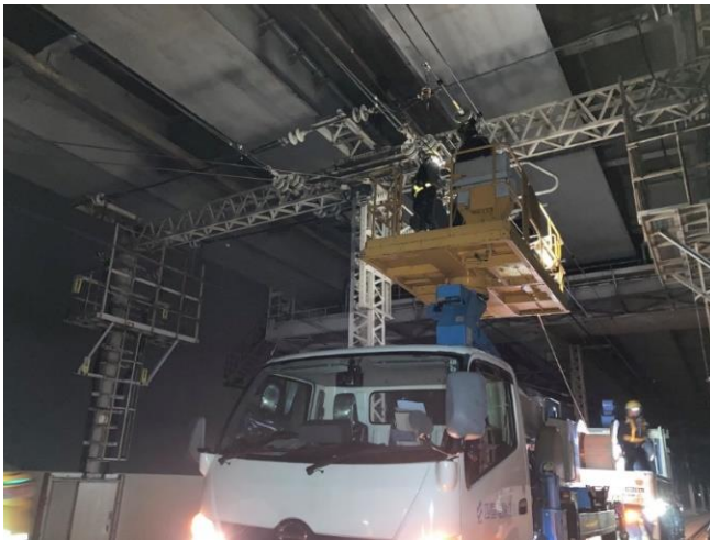
Process of installation on the Seto-Ohashi Line
