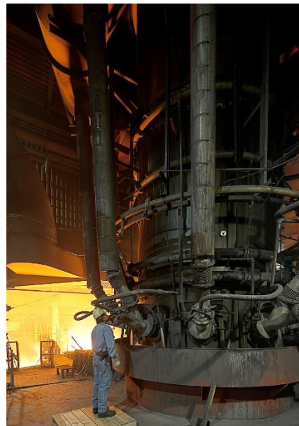
Confirming the combustion condition in the cupola furnace
