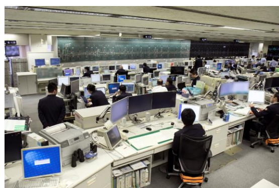
Shinkansen General Control Center
