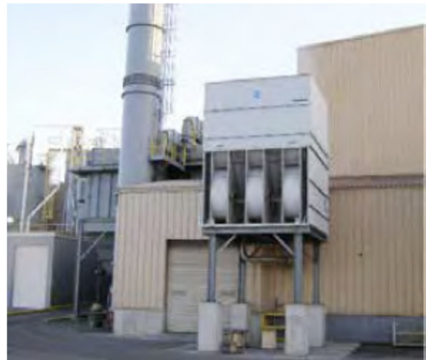
Closed-loop cooling water systems introduced at Plant 1
