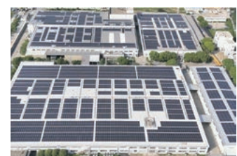
Solar power generation panels installed at Proterial Cable (Suzhou) Co., Ltd.
