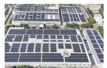
Solar power generation panels installed at Proterial Cable (Suzhou) Co., Ltd.
