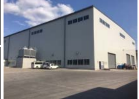
New building for structural steel castings
