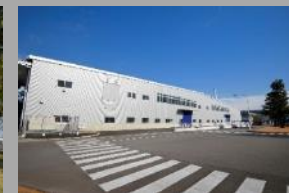
Ferrite magnets (Started operation in Feb 2018)
